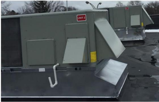
Roof top air handling units of each building shall display a 4" high minimum sign or label which consist of white reflective letters on a red background, and shall be permanently attached, at normal eye level on the roof top or air handling unit. The numbering of these units shall correspond with the FACP address.
