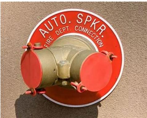
NFPA 13 – Section 8.17.2.4.5 Where a fire department connection services only a portion of a building, a sign shall be attached indicating the portions of the building served.
